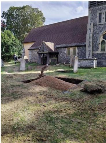
The first phases of the church works were completed just before Christmas. During this phase, the drainage system has been re-designed to take water well away from the walls of the church. Two large soakaways were created and the guttering around the church and hall was replaced.
